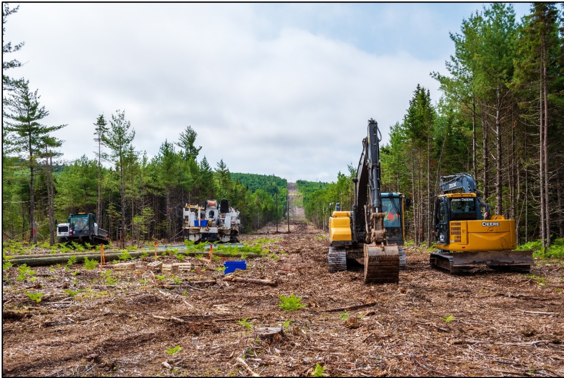
Figure 23: Area at Structure 18, facing south.
