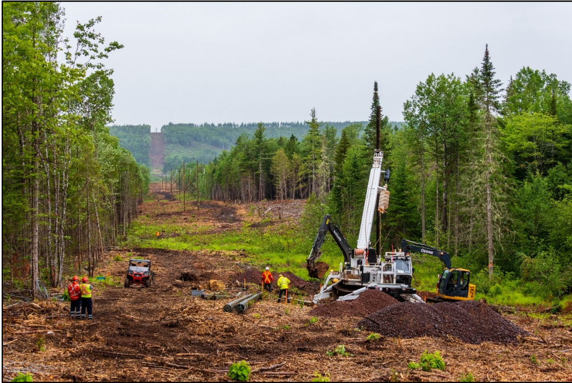
Figure 19: Structure 13, facing north.
