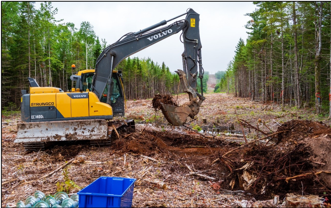
Figure 21: Structure 17, facing north.
