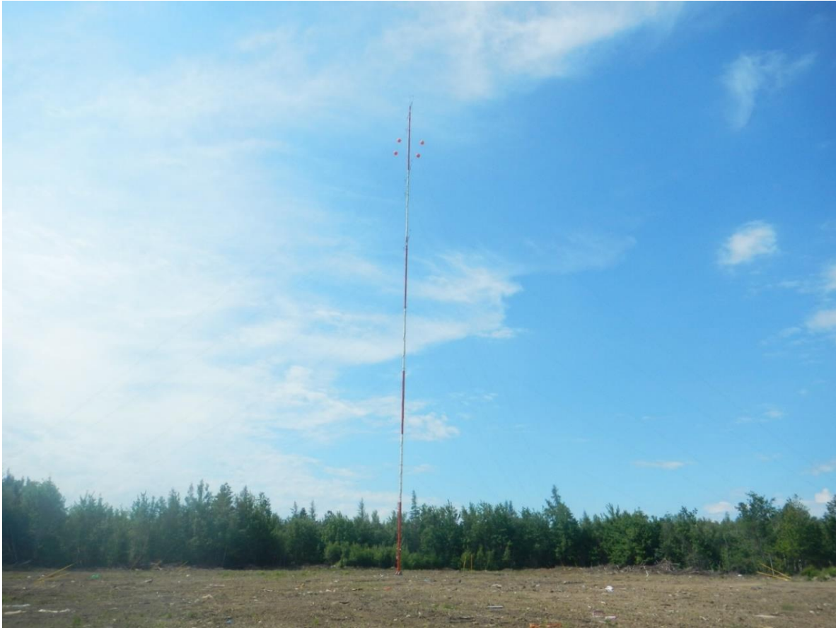
Figure 4-4: The 60m Met Tower installed in May 2017
