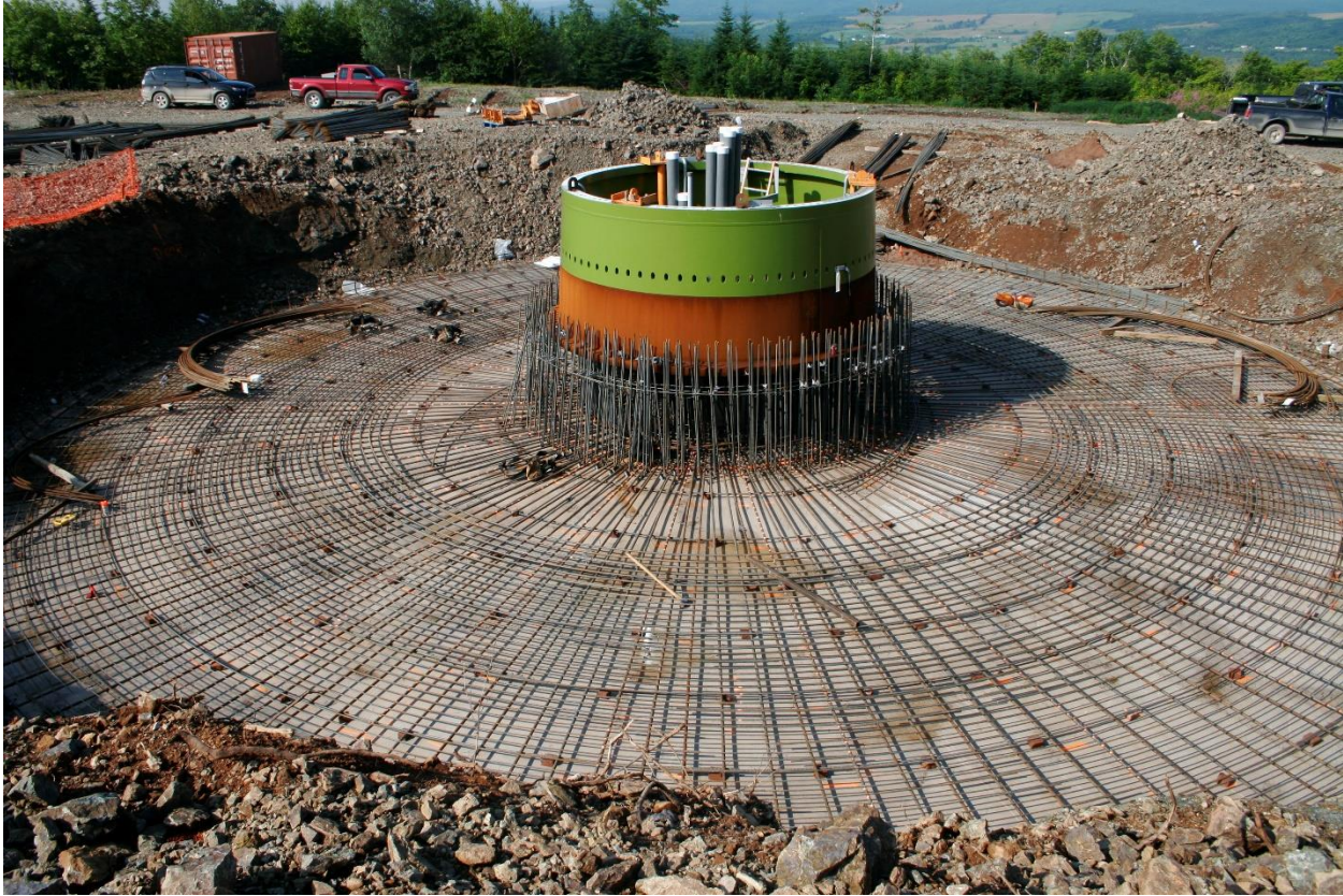
Figure 2-5: Construction of a concrete foundation at Natural Forces' Fairmont Wind Farm.
