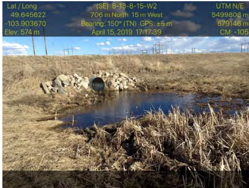
Photo 3.4-2 Standing water at culvert site within Project Area. Taken on April 15, 2019.
