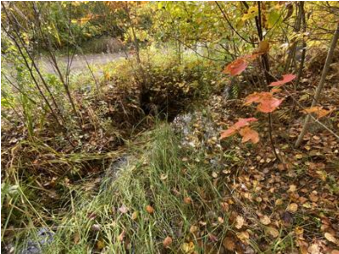
T2 October 7, 2022 at road crossing (culvert) of PDA
