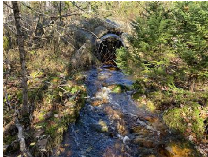
T1 October 20, 2022 at road crossing (culvert) of PDA
