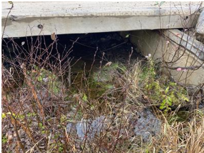
T1 November 1, 2022 at road crossing (bridge) of PDA
