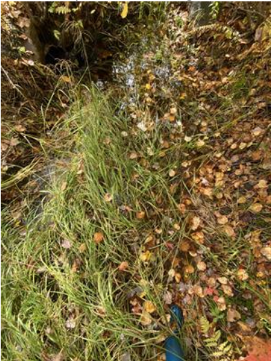
T2 October 7, 2022 at road crossing (culvert)of PDA
