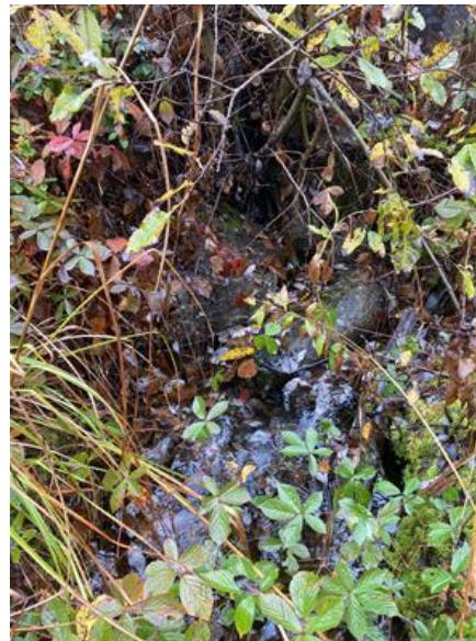
T1 October 19, 2022 raised culvert at road crossing
