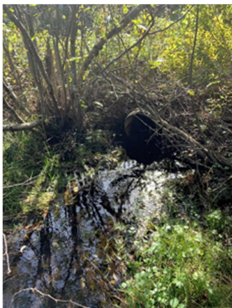
Photo 11. Culvert at outlet of Wetland 5 (5 October 2021)
