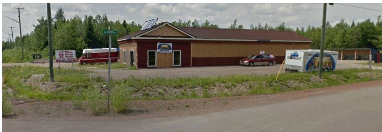
Figure 3: S & E Metal Roofing building showing few small windows that do not face the turbine location.
