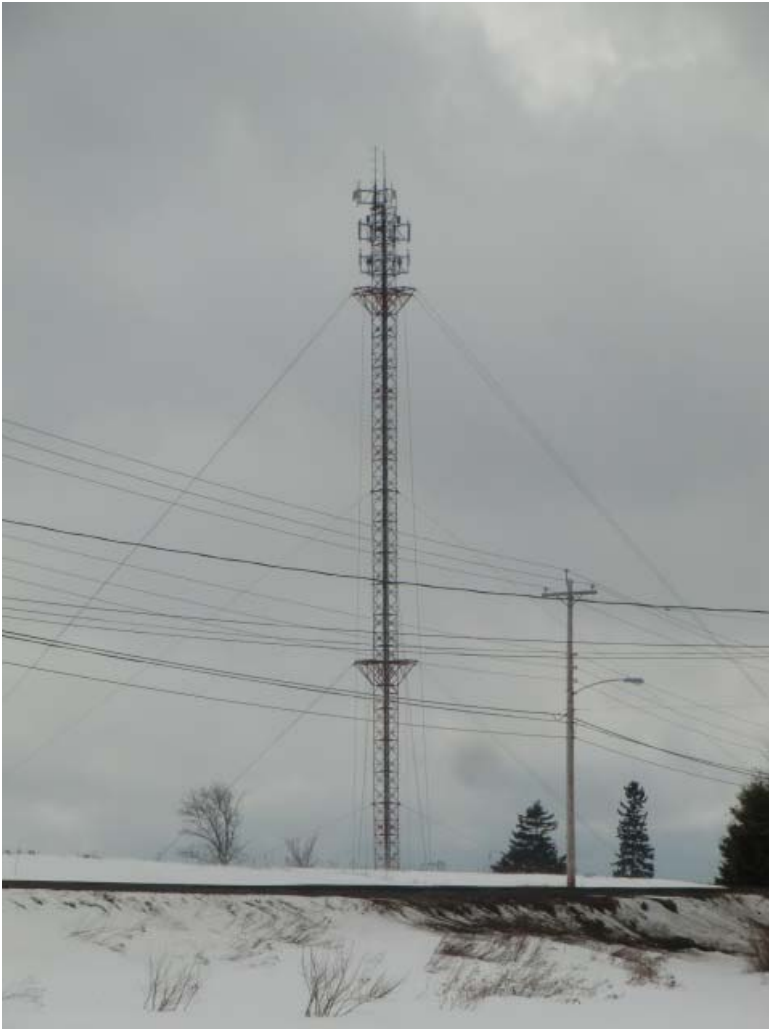
Figure 3 – Bell John Black Road Tower
